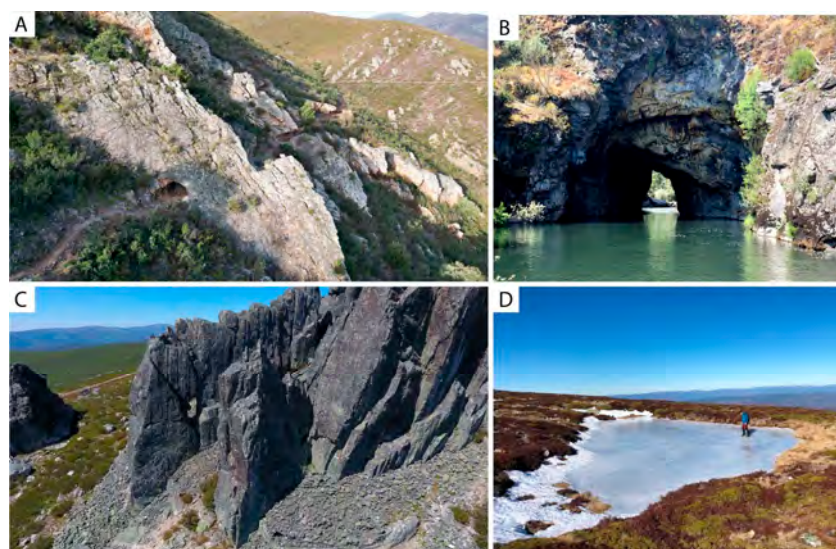
Figure 5. (A) Tunnel-canal near Pombriego. (B) Montefurado Tunnel, used for mining auriferous deposits. (C) Inter-basin transfer canal comprising an elevated tunnel, Pozos de Cabrera. (D) Snow reservoir at Sierra del Teleno.
